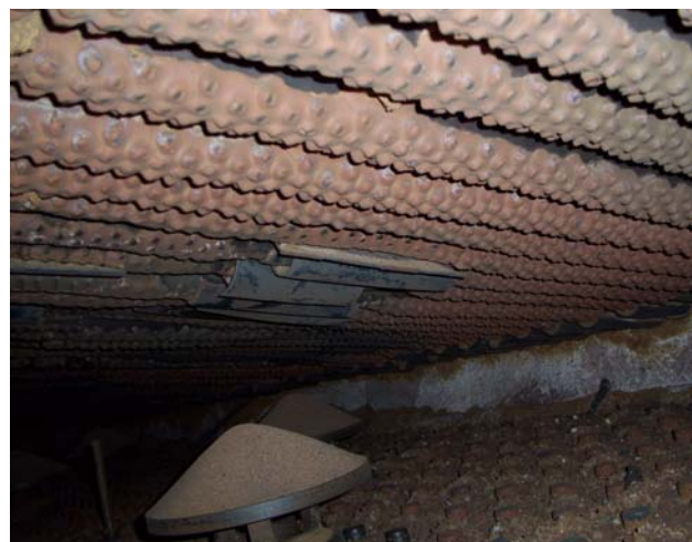
Photo 6- Fusion of ash in case of high iron.
